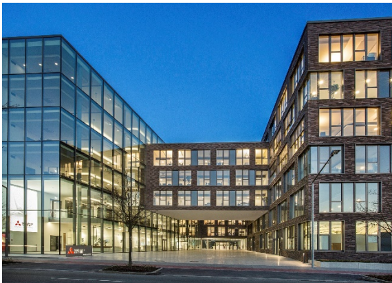
Picture 1, 2 + 3: The Factory Automation Division of Mitsubishi Electric Europe B.V. has installed an extensive range of building automation and security products in the newly built German Branch in Ratingen
